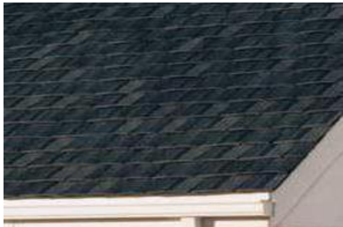
Stone-covered steel tiles are extremely fire-resistant
