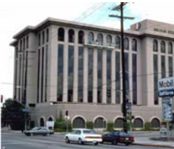
American Insurance Consultants building in Sherman Oaks (1994 Northridge Earthquake) – Joints in moment frame fractured
