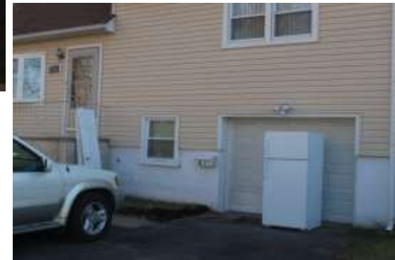
Damaged contents in garage
