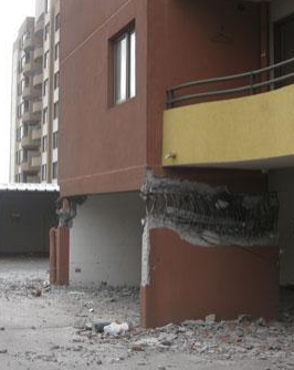
Concepcion. Edificio Centro Mayor, 17 stories. Transverse wall at second floor.
