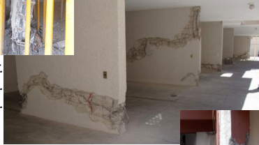
Concepcion. Edificio Centro Mayor, 17 stories. Transverse wall at second floor.
