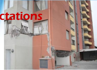
Concepcion. Edificio Centro Mayor, 17 stories. Transverse wall at second floor.
