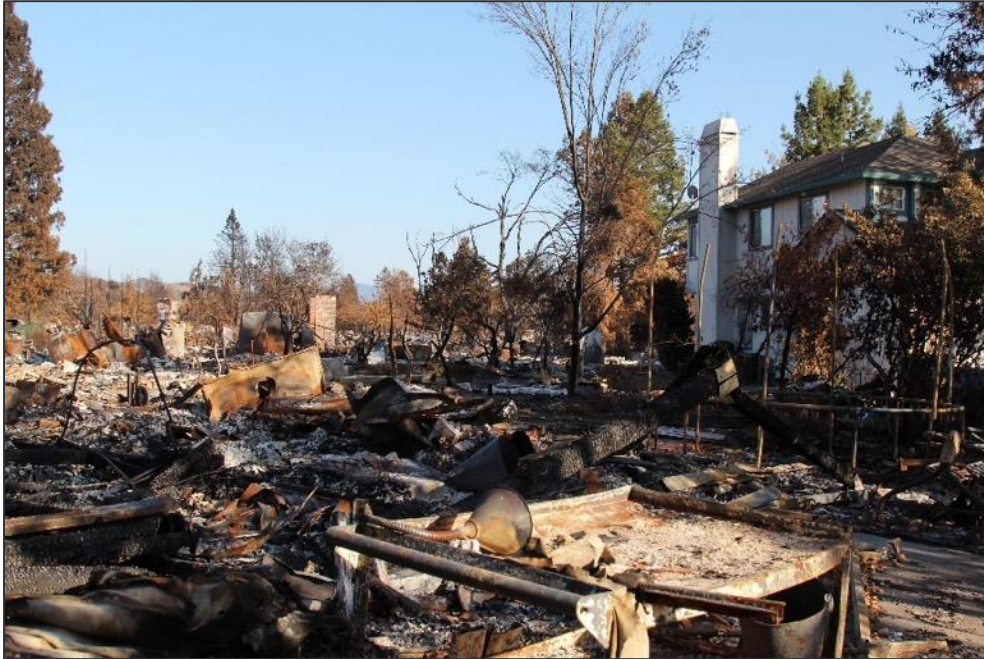
AIR Tubbs Fire Damage Survey 2017
