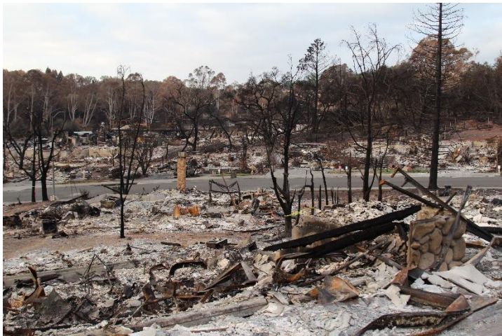
Fountain Grove, AIR Tubbs Fire Damage Survey 2017
